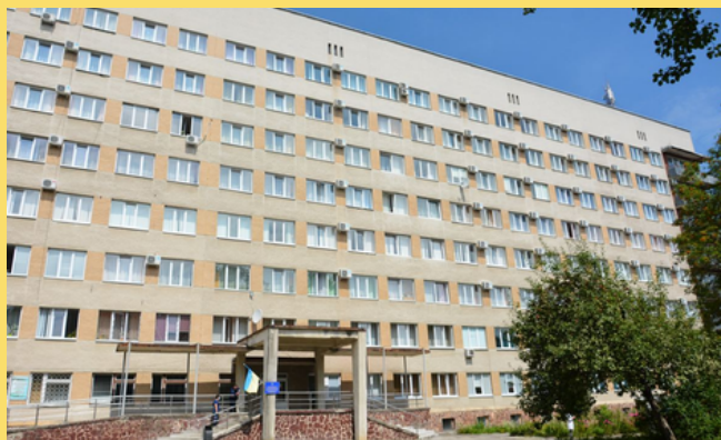
KALUSH CENTRAL DISTRICT HOSPITAL
